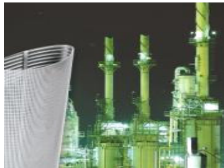
Hydrocarbon Process Industries
